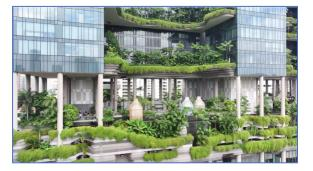
Singapore is also encouraging the integration of greenery directly into buildings by offering financial incentives for rooftop gardens and vertical green facades. The foliage works as natural blinds, shading the structure and insulating the building's material from the heat, reducing the need for air conditioning.
