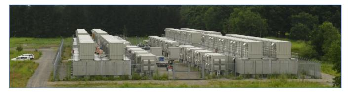
Just outside the building that houses the gleaming floor-to-ceiling tanks, Sumitomo has built a new version of its flow batteries, this time tucking all of their components into shipping containers. That makes them faster and cheaper to build than the \$100 million indoor demonstration plant next door.
