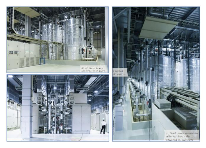
All of these tanks are lined up in pairs. One tank holds vanadium with a more positive charge, while the other tank holds vanadium with a more negative charge. Every tank is hooked up to a set of pipes that pump the vanadium into battery cells stacked in cabinets on the second floor. Vanadium flows through each battery cell on either side of a membrane — which is why it's called a flow battery.
